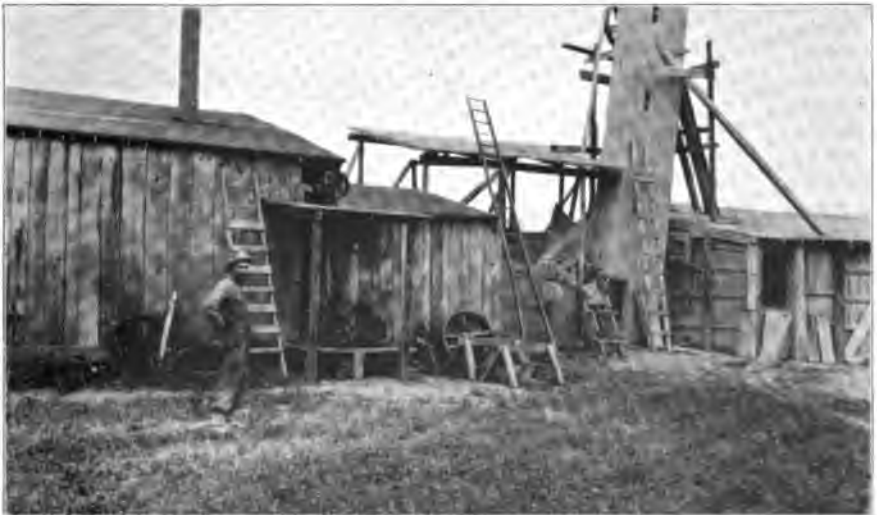
B.—Limestone crusher north of Munser Knob preparing agricultural limestone.
